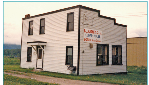
The office of B.J. Carney Pole & Co. Ltd. at 709 Vernon Street in 1980. [edms 3201]
